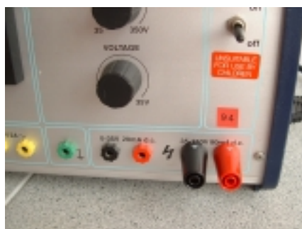
Figure 2 Showing fitment of 4 mm shrouded connectors over unshrouded socket outlets.
